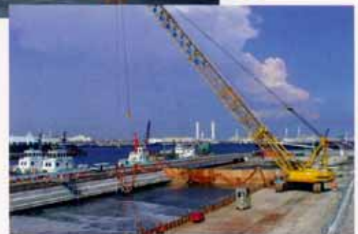
Material Being Placed
